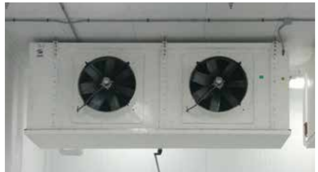
Top: A standard 50 TR RDC unit can be charged with 75 lbm from an ammonia cylinder in as little as 15 minutes Bottom: DX evaporators
