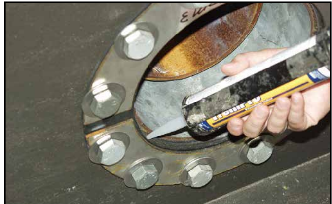
Figure 54 – Caulk Exposed Galvanized Steel
