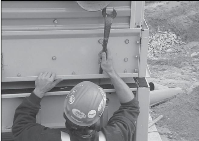
Figure 5 – Drift Pin Alignment
