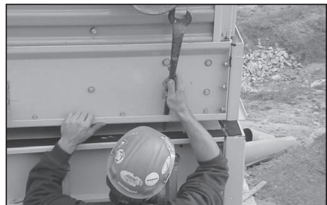
Figure 5 – Section Alignment Using Drift Pins
