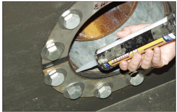
Figure 16 – Caulk Exposed Galvanized Steel
